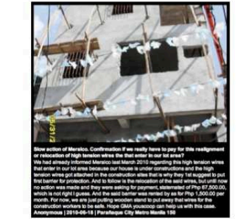
New action of Marikina. Contractors if we really have to pay for this realignment or relocation of high tension wires that that enter in our lot area? We had already informed Marikina and Metro 2010 regarding this high tension wires that enter in our lot area because our house is under construction and the high tension wires got attached in the construction site that is why they let us get to find barrier for protection. And it below is the installation of the said wires, but still now no action was made and they were asking for payment, estimated of P10,000.00 per month. For now, we are just putting wooden stand to put away that wires for the construction workers to be safe. Hope GMA7 producers will help us with this case. Anonymous | 2010-06-15 | Paraiso City Metro Manila 150
