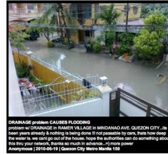
DRAINAGE problem CAUSES FLOODING problem w/ DRAINAGE in RAMER VILLAGE in MINDANAO AVE. QUEZON CITY... Anonymous | 2010-06-19 | Quezon City Metro Manila 150
